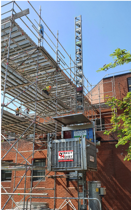
Direct Hoist's GEDA 500Z ZP/850, a transport platform, can carry 850kg goods and materials.
