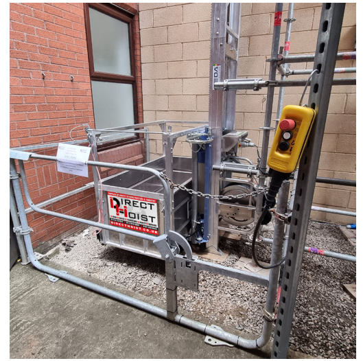
GEDA 200 ladder, with a lifting capacity of 200kg is a goods-only hoist for tools and materials.
