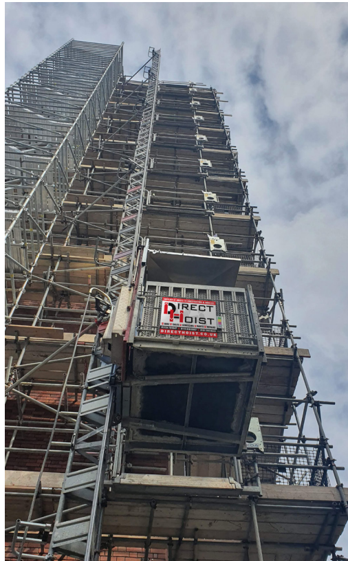
GEDA 500Z ZP/850 is capable of being installed 100m high while carrying five people or 850kg.
