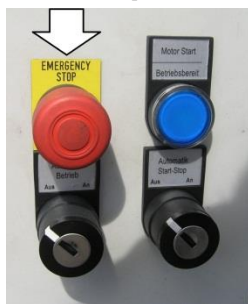
Fig. 13: EMERGENCY STOP button (arrow) at the switch cabinet
